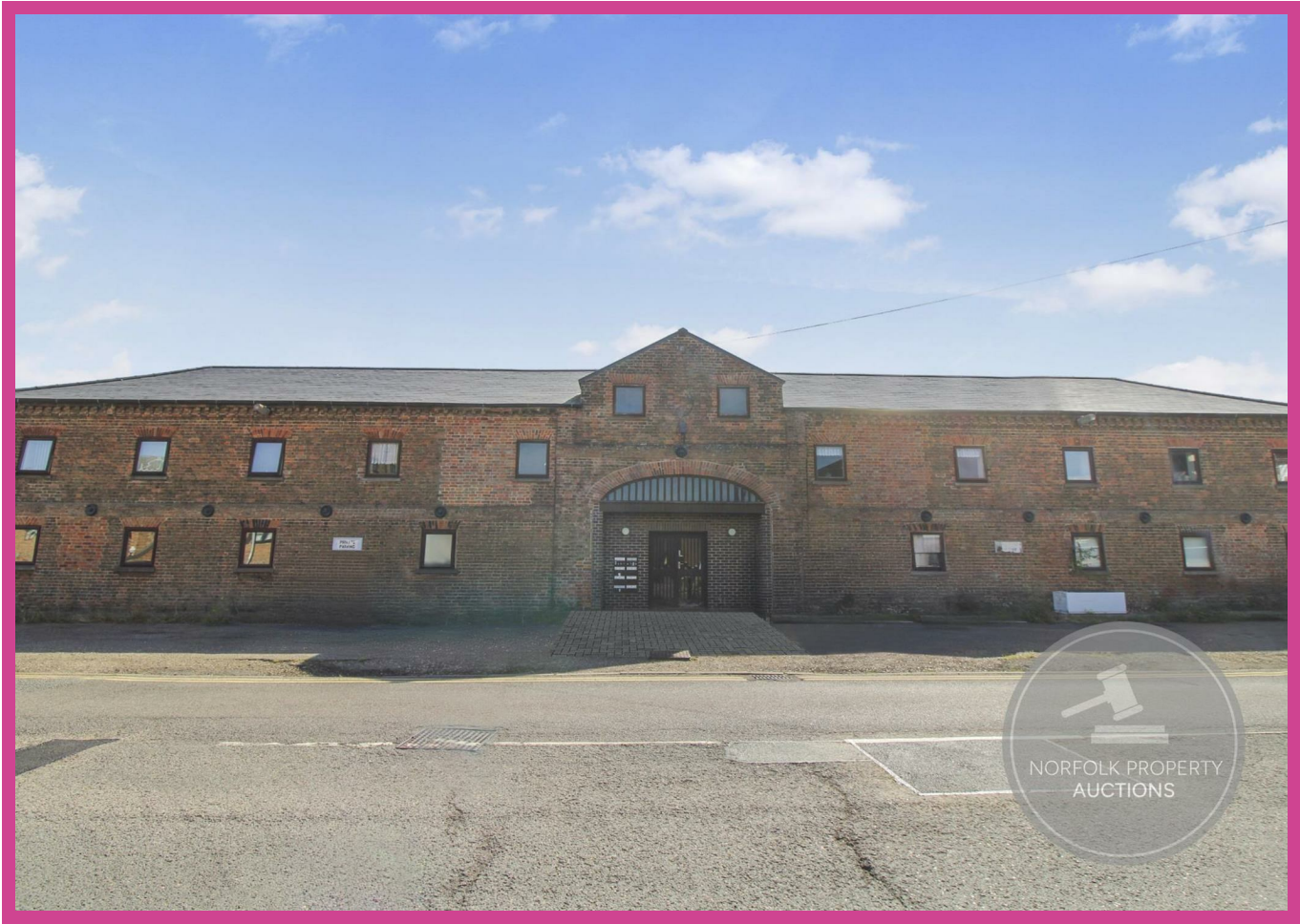
West Bank Sutton Bridge Spalding PE12 9TU
